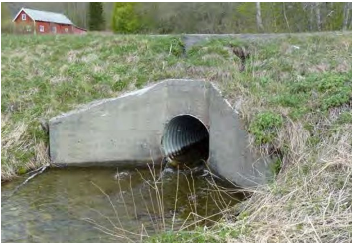
Figure 7 Example of V-shaped culvert intake.
