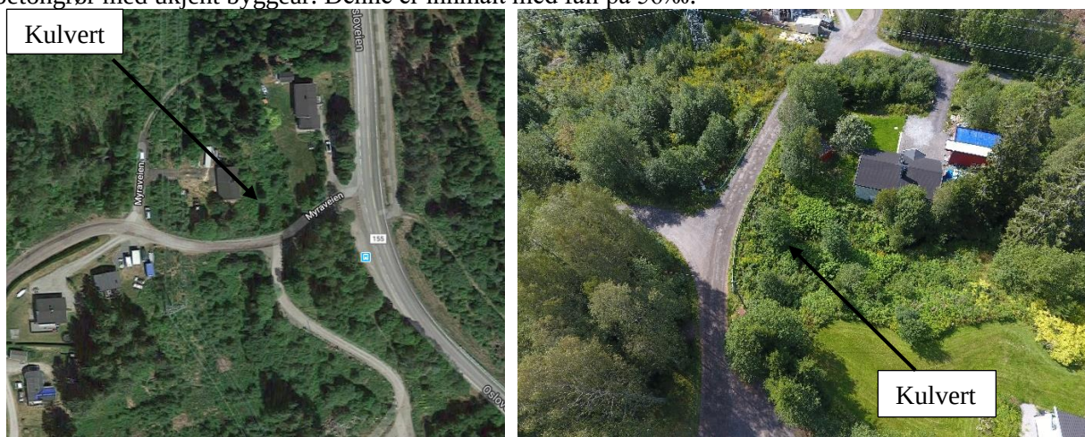
Figur 11: Kulvert under Myraveien
